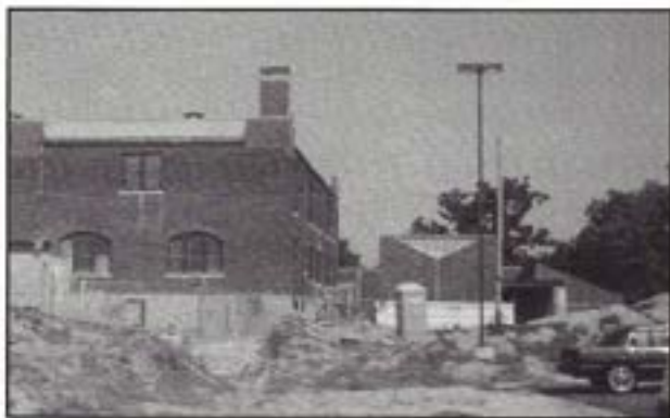
All Saints School. Construction of Gymnasium. 1989
