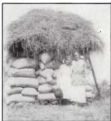
Sacks of wheat after threshing. Protected by a shed made of posts in ground covered by a thatch roof. Courtesy of H. Iffrig
