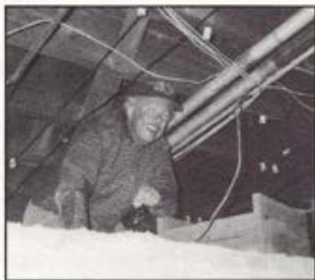
Father Henning inspecting church basement crawl area, 1997
