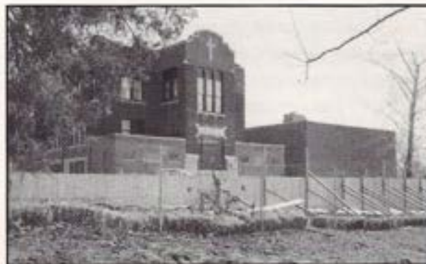
All Saints School. Construction of Parish Center. 1989
