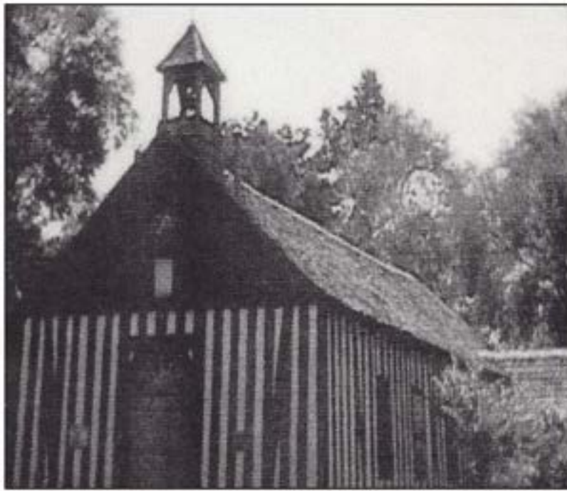
Holy Family Church, Cahokia, Illinois, built in the French style (with vertical logs). Our first parish church was said to be in this style, similar, but smaller.
