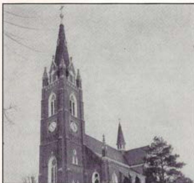
Church Tower, completed in 1916.
